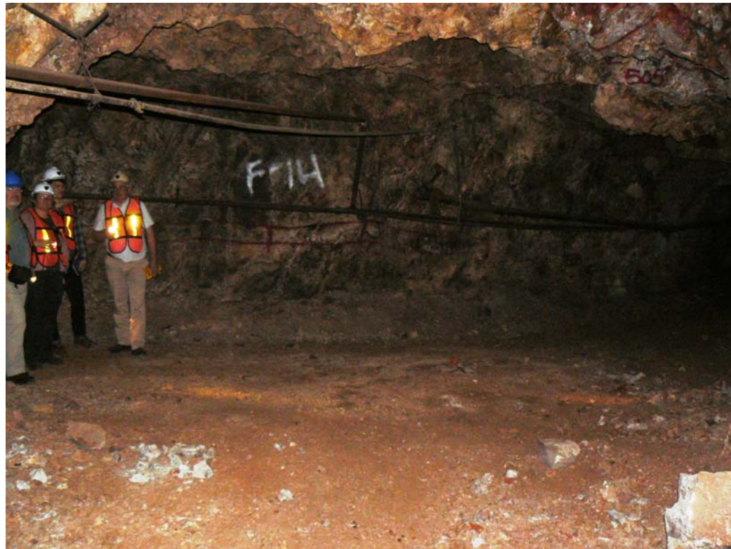
Figure 16: A General View, Looking Approximately West) of the Large Span Intersection Area Where A Crosscut Meets the Adundancia Vein Drift (note the lack of any support and the limited amount fallen material on the footwall of the drift) (taken during AMEC's early January 2012 site visit)
